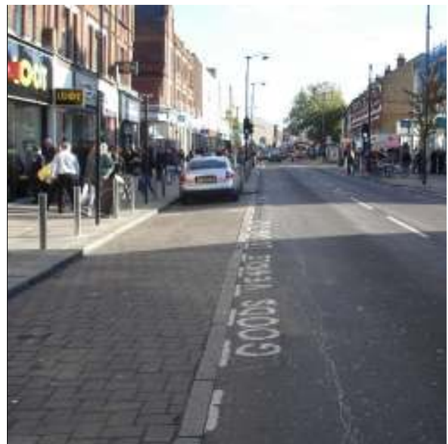
Existing High Road loading bay
