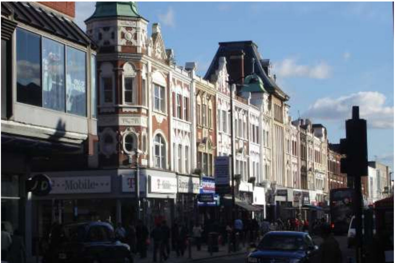
Cheapside buildings, Wood Green High Road
