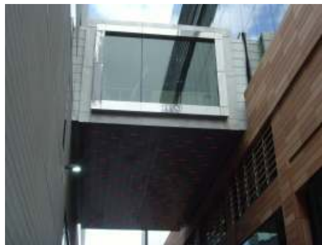
Good practice image: Link bridge in new commercial development, Liverpool One
