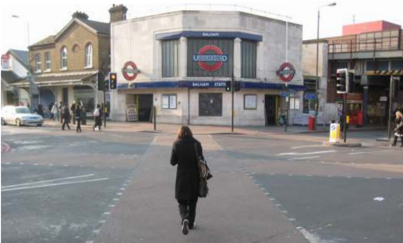
Good practice image: diagonal pedestrian crossing, Balham Station, London
