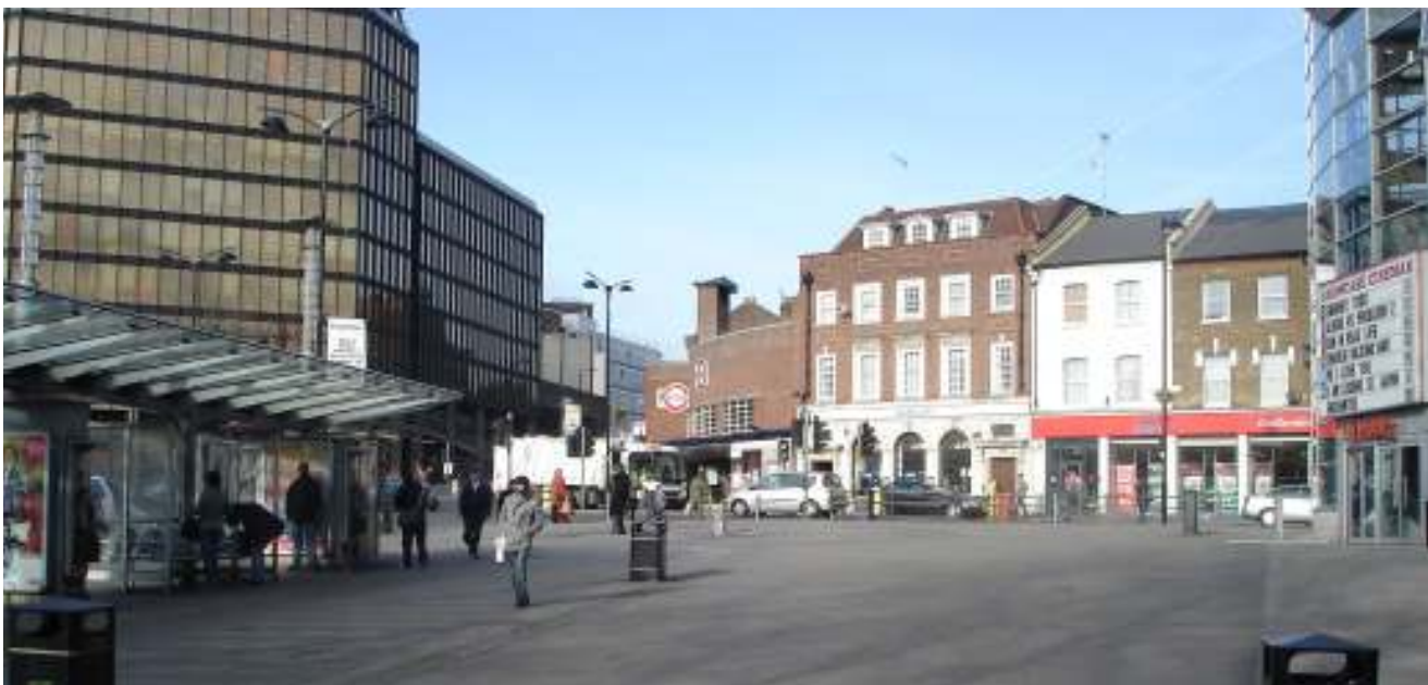
The Broadway, looking north towards Wood Green tube station and River Park House
