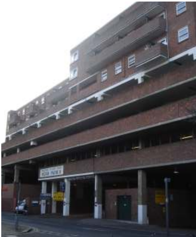
Bury Road Car Park
