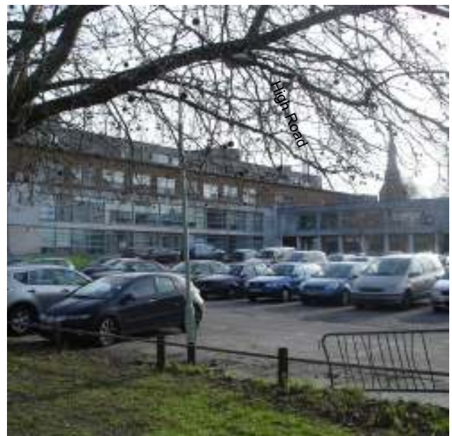
Civic Centre and car park
